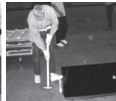
Always tap the panel into place with the pounding block. NEVER hit the metal edge with a sledgehammer, since it will damage the metal tongue.
