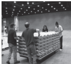
Handling panels (four people per panel). Lift the panels one by one and avoid sliding them, since it will scratch the finish.
