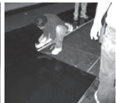
Fix B1 to A1 and slide it into row A while keeping row A on the chalk line to ensure alignment.
