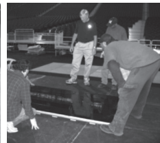
Set the first panel (A1) at the determined starting point to begin court installation.
